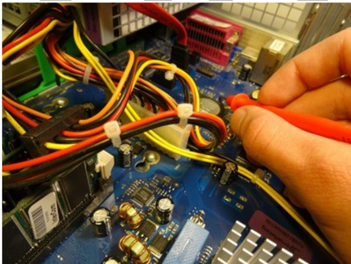
Figure 5 High Voltage Wire Example
